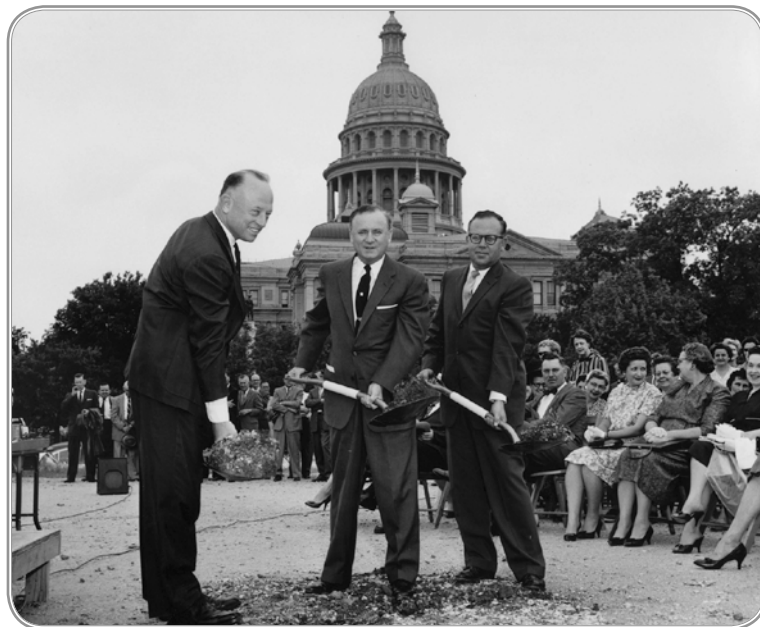
Governor Daniel, center breaking ground for the Zavala Building.
